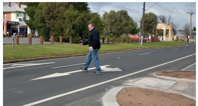
Councillor Ron Eason making use of one of the new crossing points in Avoca's High Street that are under construction.
