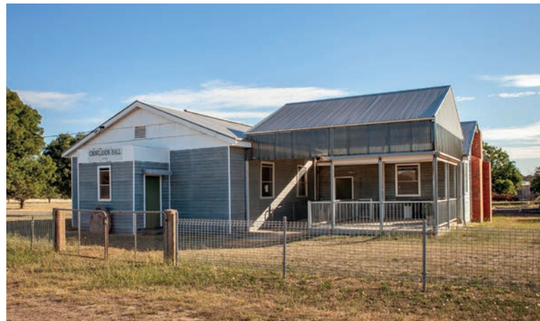
The Crowlands Hall and Reserves Committee was awarded $5400 as part of the Community Grants Program to install kitchen split systems.
