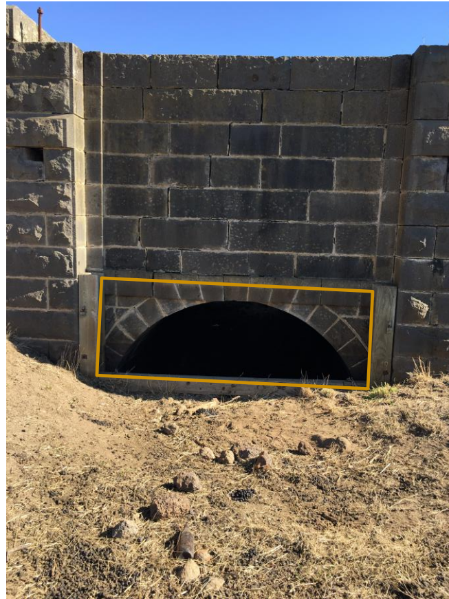
FIGURE 5-17 PICTURE OF THE BRIDGE AT LAKE GOLDSMITH DIVERSION CHANNEL
