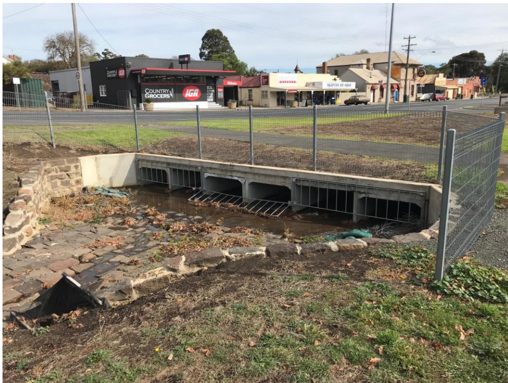
FIGURE 4-2 UPGRADED MITIGATION CULVERTS IN MONTGOMERY STREET, SKIPTON
