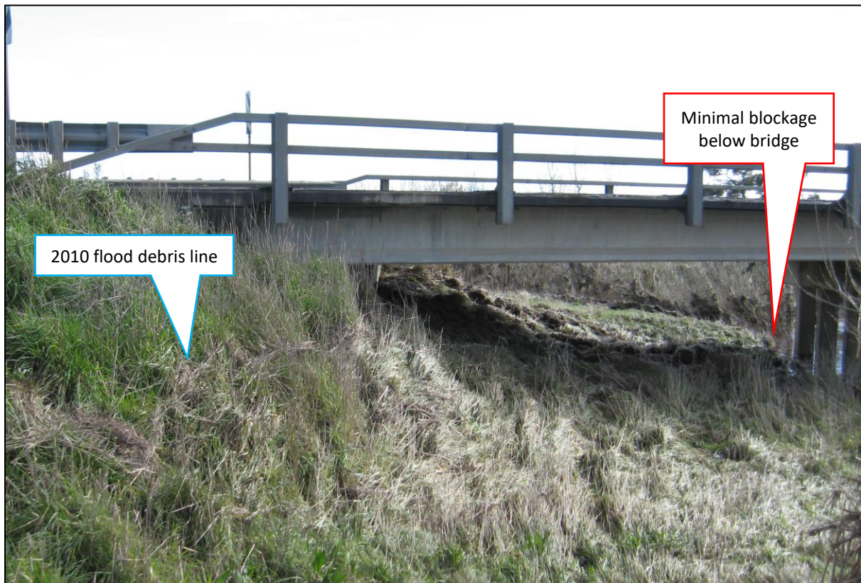
Plate 1 - Photograph of part section of the Western Highway bridge that was taken following the 2010 flood showing minimal debris/blockage
