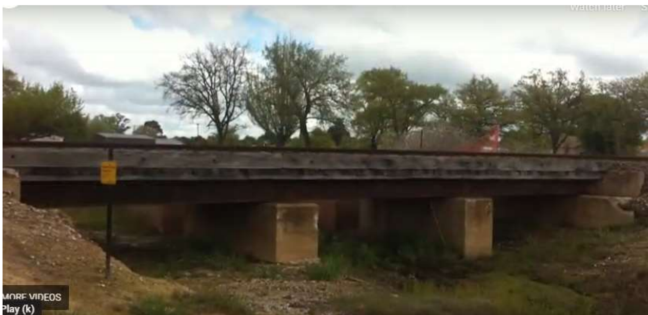
Beaufort railway embankment drainage before the mitigation works (VicTrack).
