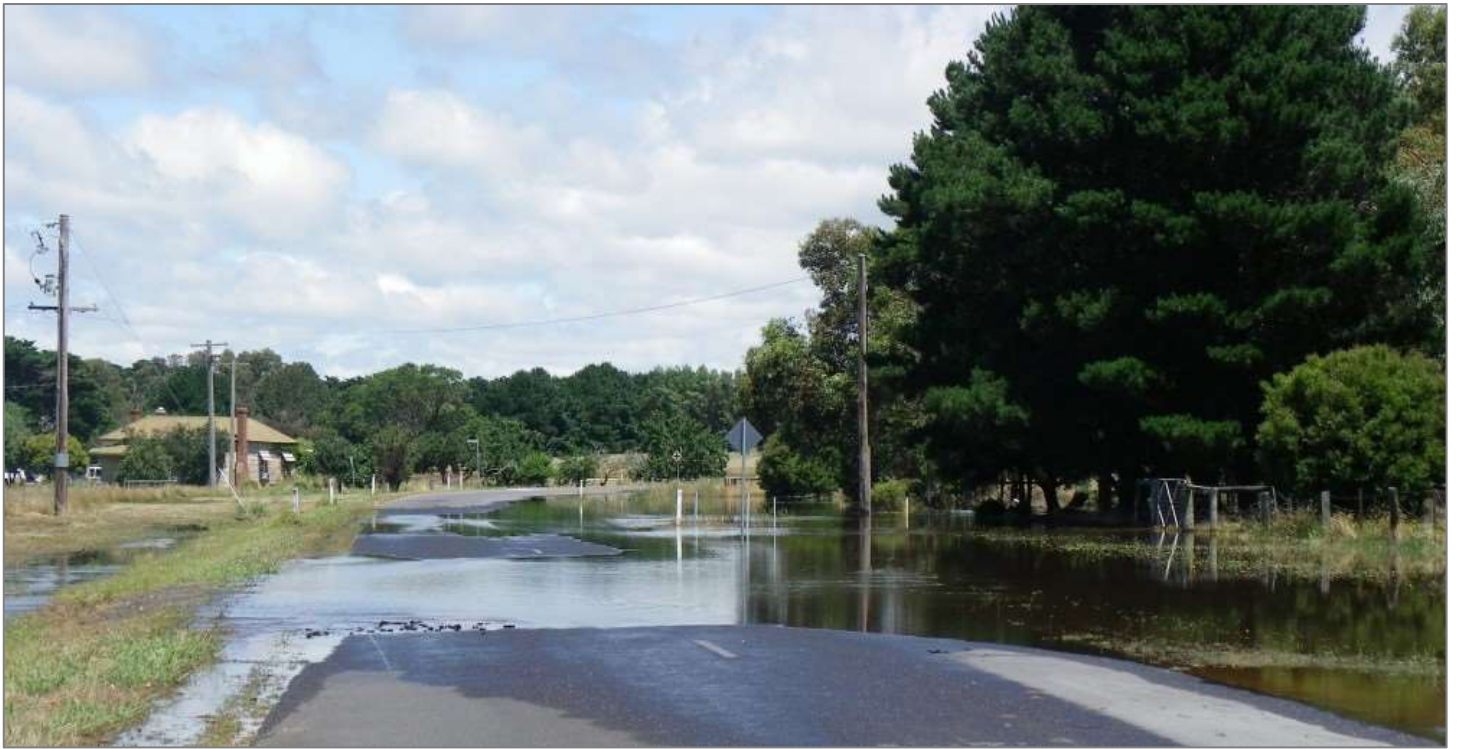
Flooding across the Fiery Creek Bridge, Raglan during the January 2011 flood event (source: Lorraine Thomson).
