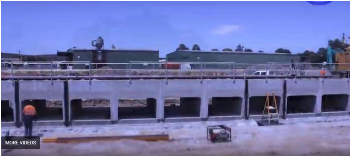
Beaufort railway embankment drainage, expanded to a 25m section of nine culverts (VicTrack).
