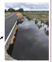
A second application has also been approved to repair rutting on road shoulders. Vehicles travel at higher speeds on these roads and have to move to the edge to pass another vehicle as the seal is narrower.
