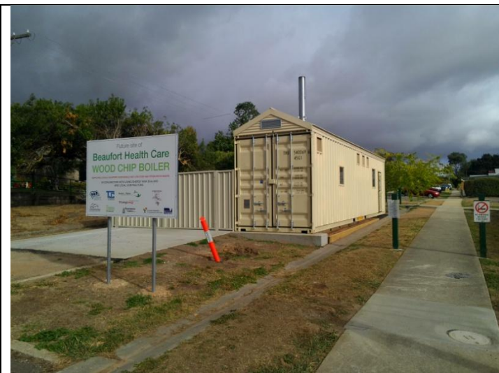
The completed boiler house
