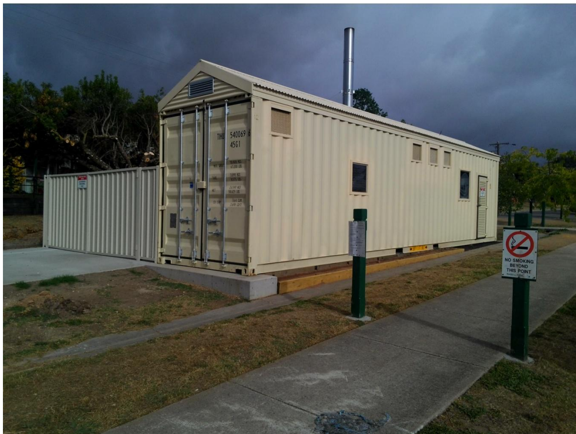
Figure 2: Boiler house and fuel store
