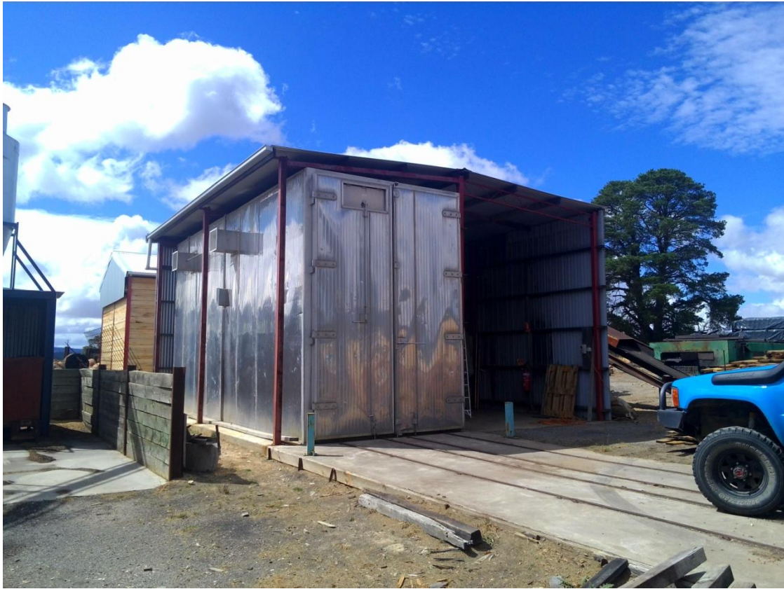
Figure 5: Photo of the timber kiln
