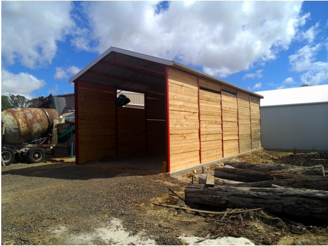
Figure 3: Photo of the chip storage shed
