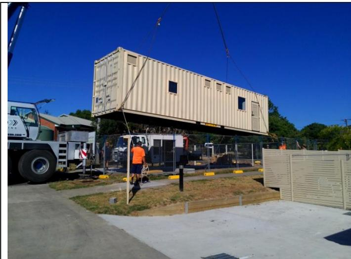
The boiler house being lowered into position
