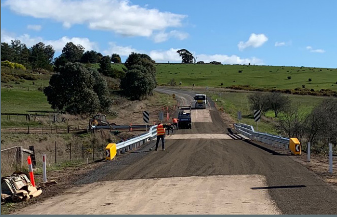
Bridge 13 on the Beaufort-Carngham Road has been replaced.
