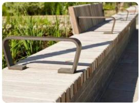
4.2 Seating on top of retaining/ seating wall
