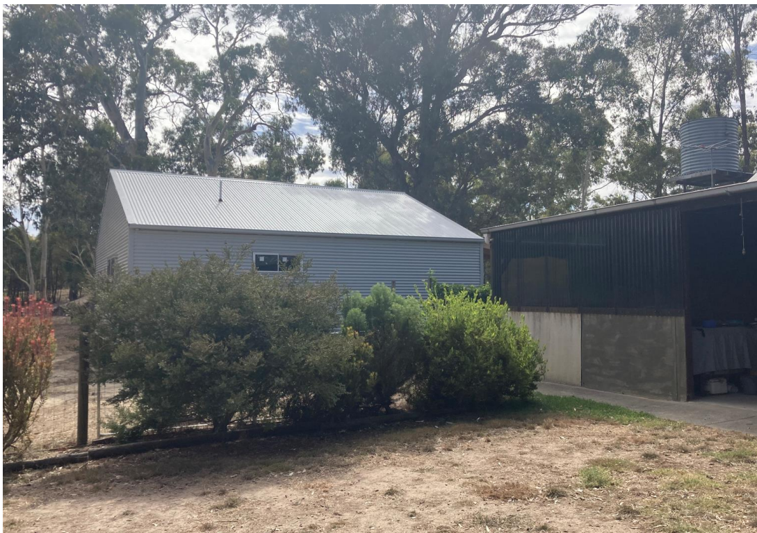
Image 7 – view of second dwelling from site entrance
