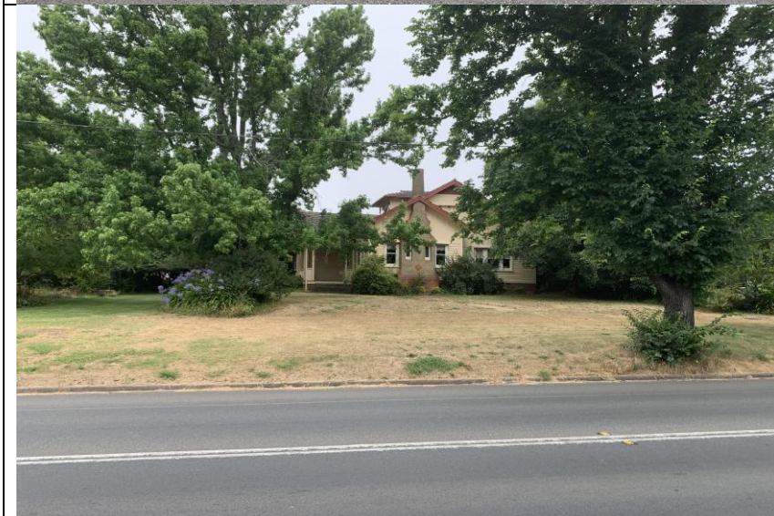
Dwelling at 1-3 Neill Street.
