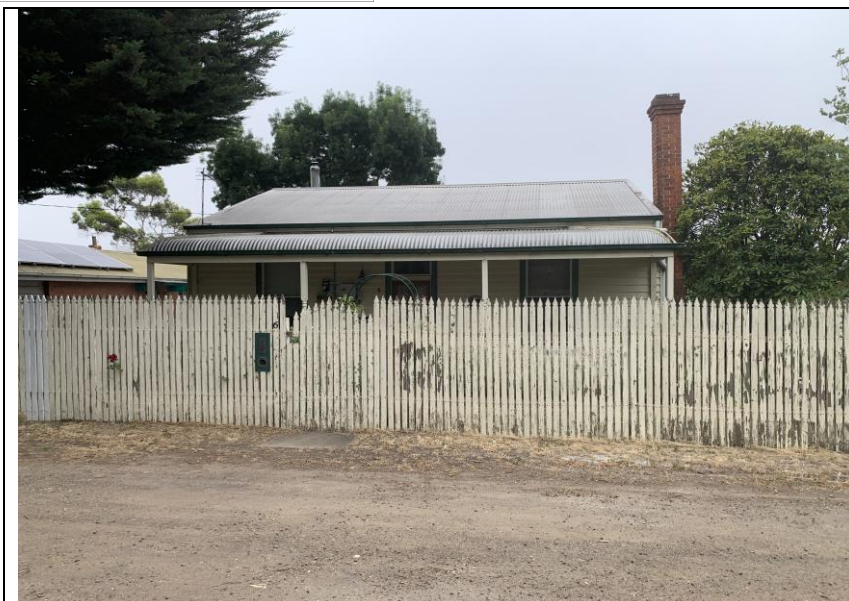
Dwelling at 6 Neill Street.
