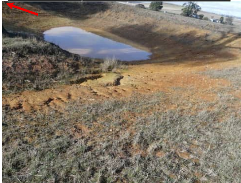
Image 21 Design spillway to the lowest point of the dam and dig a channel to form a twisting line to the low point near the fence as noted in these images.
