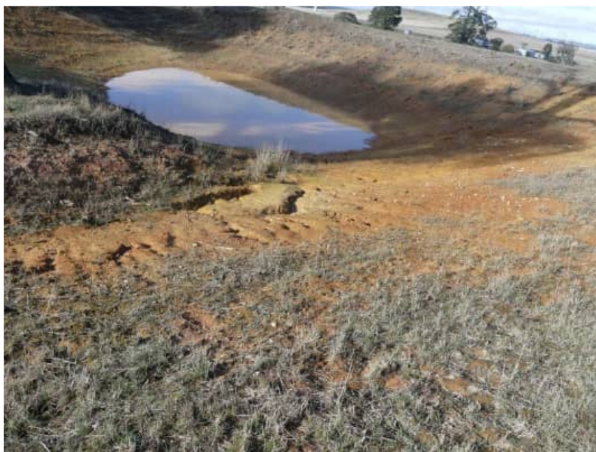
Image 46 Soil movement above the dam (south end below proposed dwelling)
