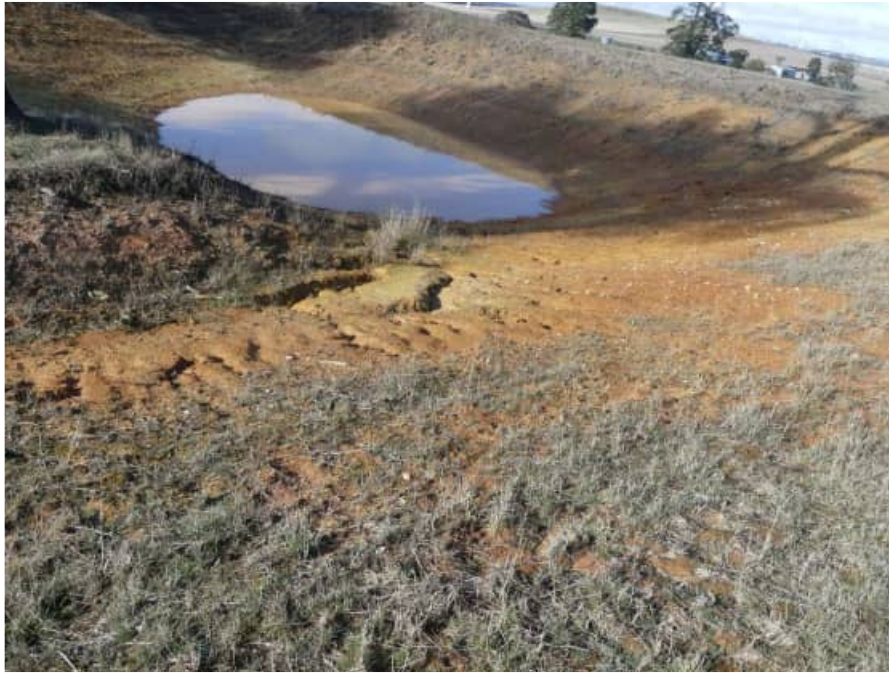
Image 9 Rill erosion of the dam from water
