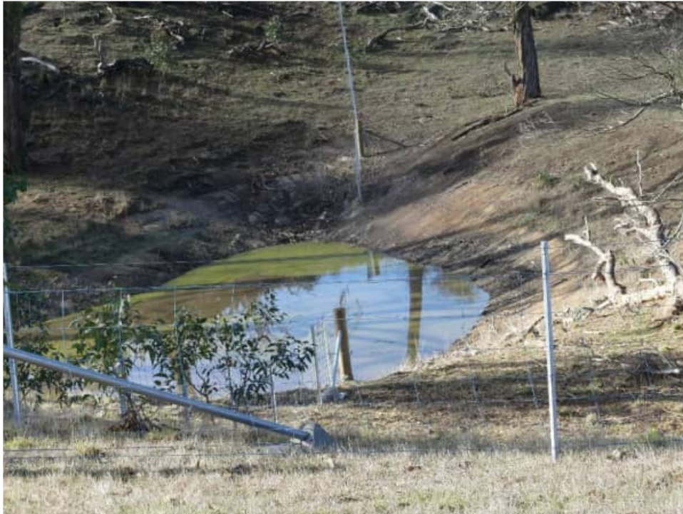
Image 11 Erosion along the edge of the dam most likely from stock.
