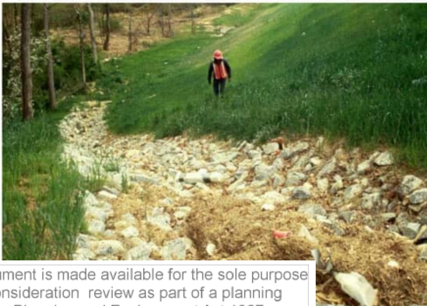
Image. 19 Rock chute to the end of the drainage line in Paddock.10
