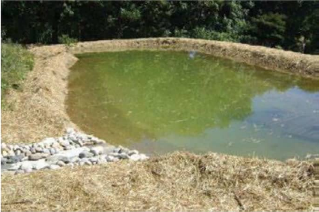
Image 22 Example of a rock spillway to the lowest point in the dam so that water flow out in extreme storm is controlled and does not continue to erode (Source: Proagrimedia, 2022)
