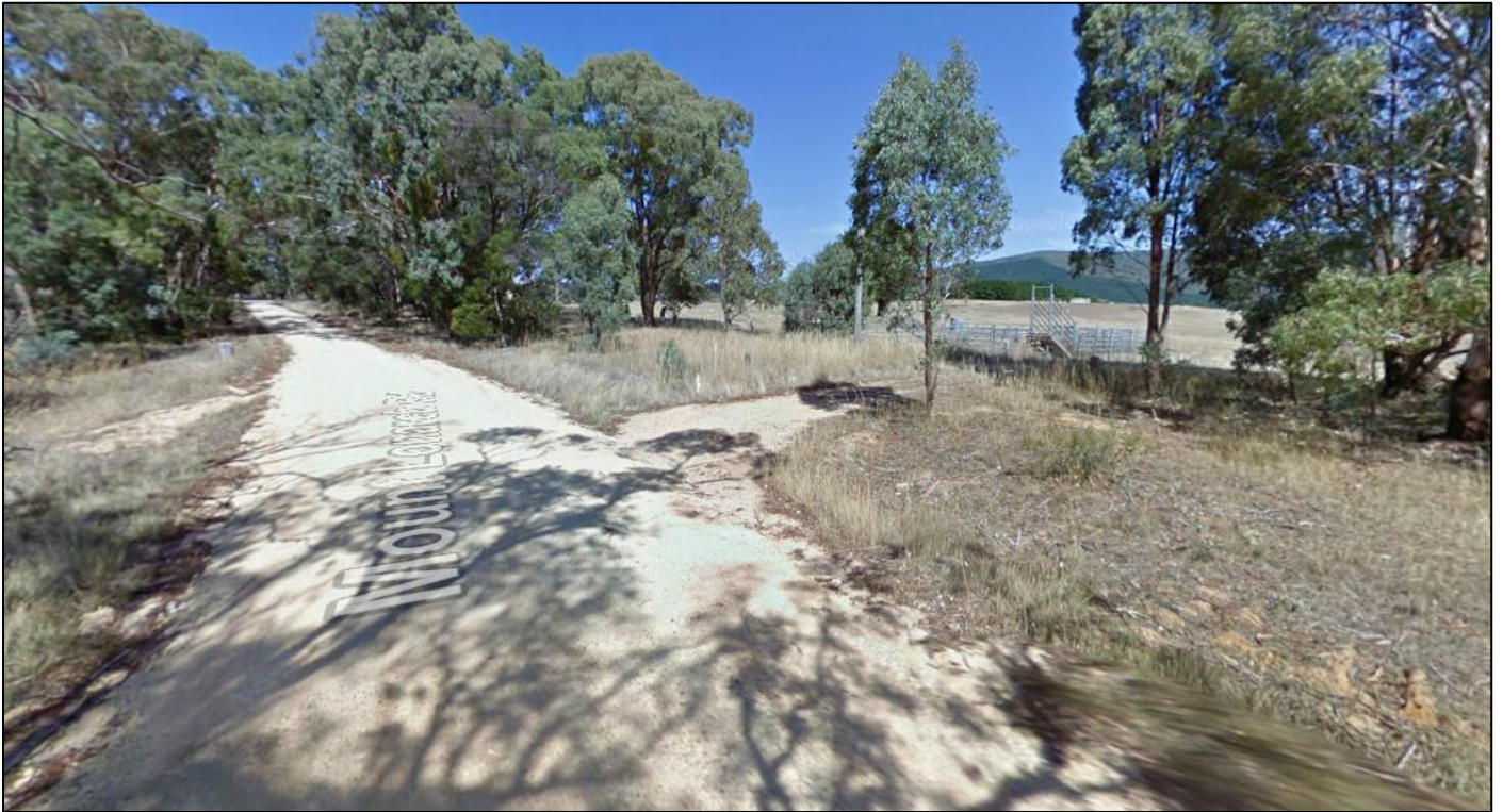
Figure 5 Roadside elevation and existing access
