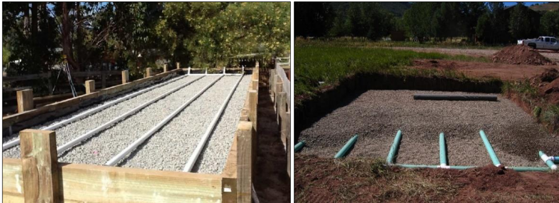
Figures 52-53 – Above and below-ground Sand Filter systems (Source: Murray Valley Septics 2019, William Kromer 2016).
