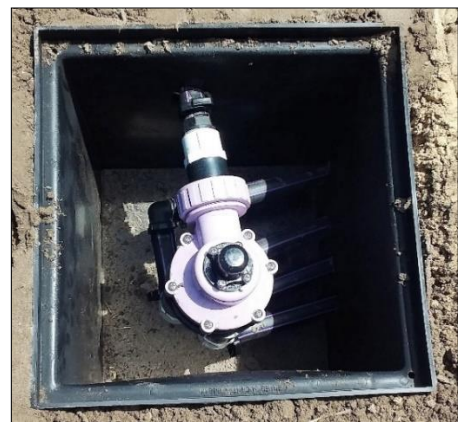
Figures 35-36 - Cross-section of soil absorption trench; Rotavale for dosing disposal areas (Source: ASNZ1547).
