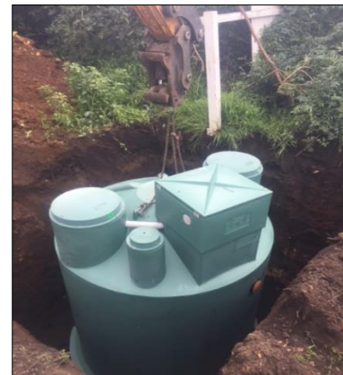
Figures 26-27 – Cross-sectional view of an aerated wastewater treatment system (AWTS); Aerated Wastewater Treatment System (Source: EHPA, Ozzikleen 2017).
