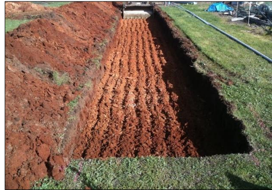
Figures 49-50 – ETA-trench/bed cross-section and site preparation (Source: ASNZS 1547 2018).
