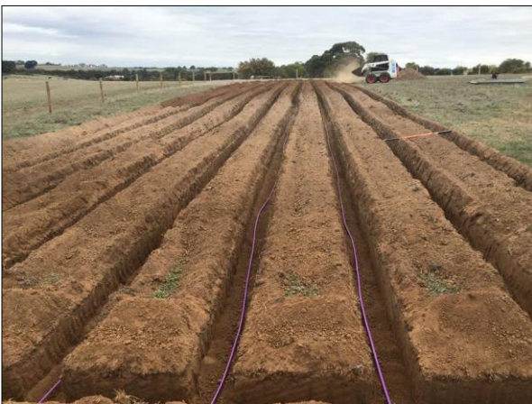
Figures 33-34 -Subsurface irrigation site preparation; ETA trenching on sloping ground (Source: ASNZ1547).
