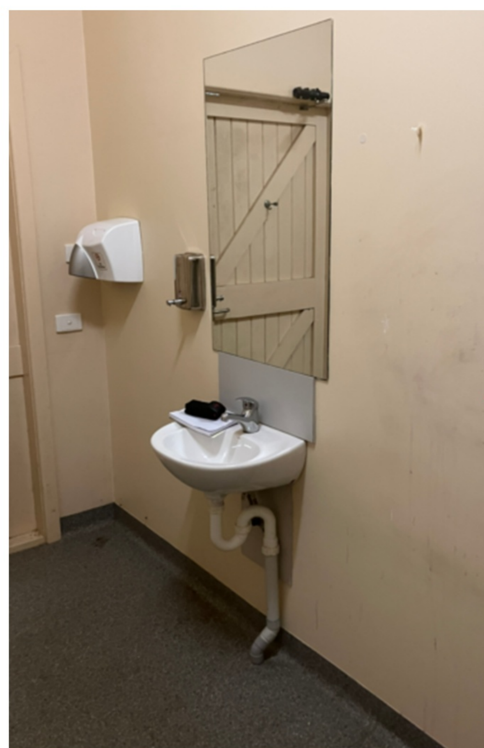
Dated wash basin and other fixtures
