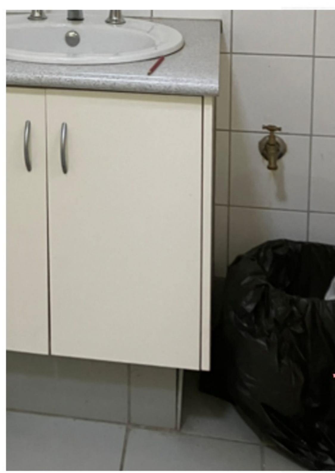
Tiles lifting under cabinetry
