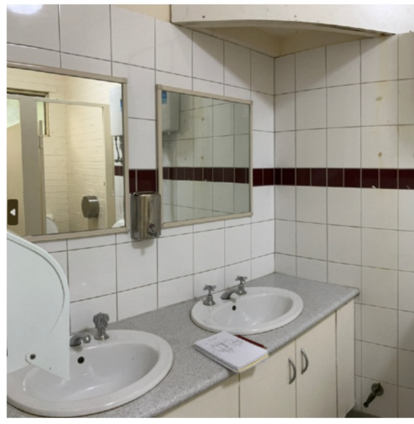
d. Mismatched mixer taps, dated drier and laminate peeling from cabinetry doors
