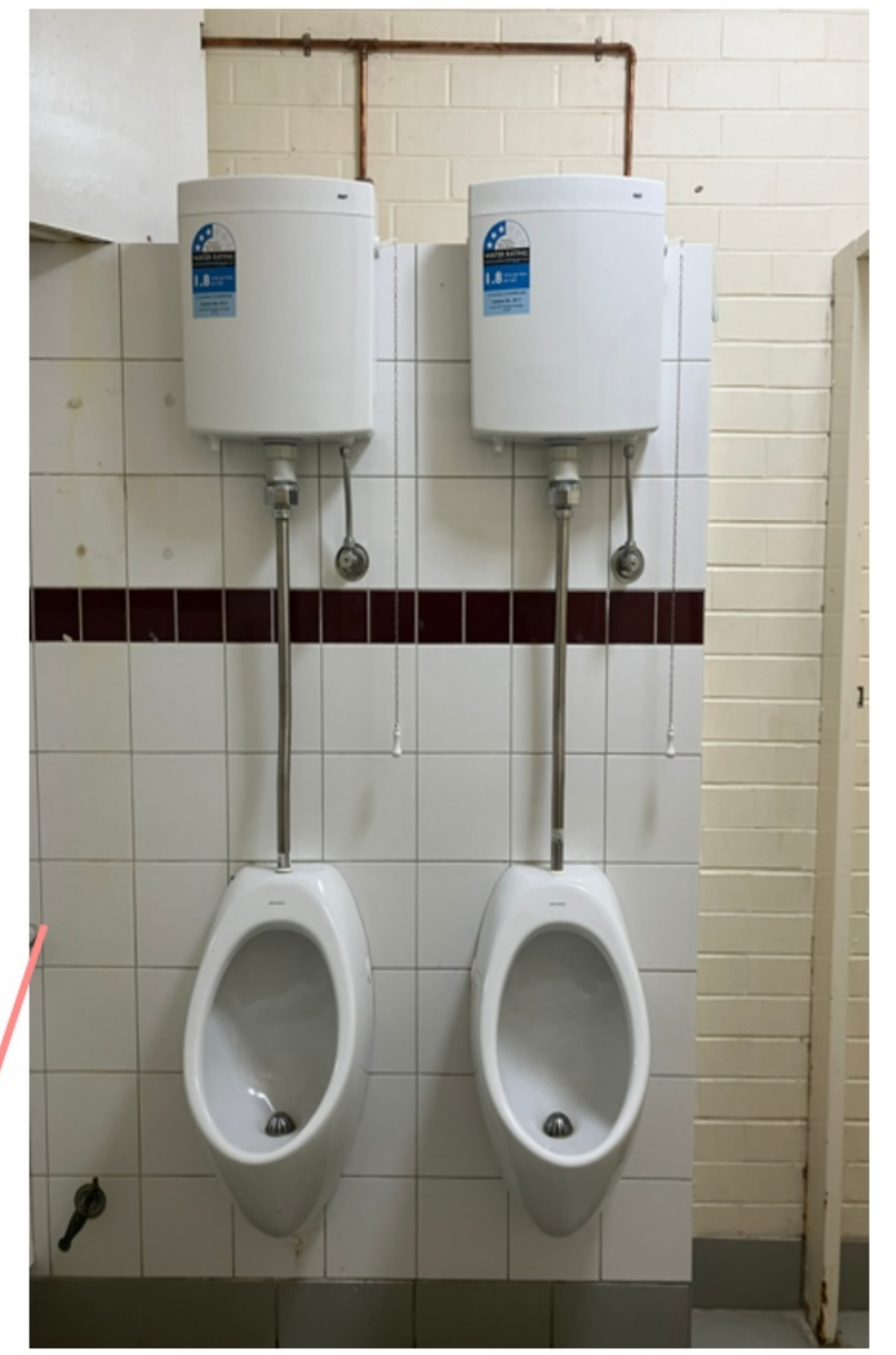
f. Urinals: Good condition, pull chain flush with exposed pipe, discolored tiles
