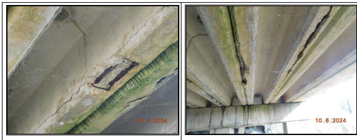
6.1.1 Back Cemetery Rd - Twin span full RC U-Slab Bridge ID 007 Condition 8
